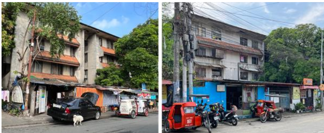
Figure 37:—Sikatuna BLISS - informal additions
