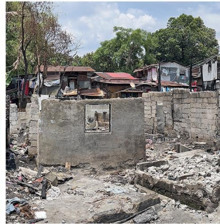
Aftermath of the fire
